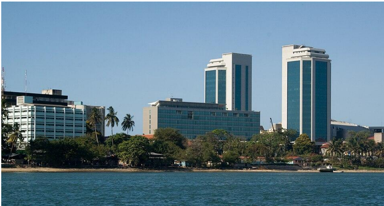
Bank of Tanzania headquarters, Dar es Salaam. Photograph: Fanny Schertzer / Wikimedia Commons, CC BY 2.5.
